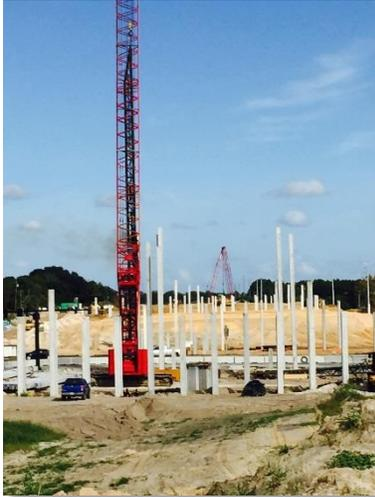
Work started on these two sections after approximately 300 gopher tortoises were relocated to a state approved recipient site per the project environmental permit. The scale of the construction is impressive. Section 1A, for example, in late 2015 was in the process of installing 700 concrete bridge piers and more than 1 million cubic yards of embankment for the elevated parkway.
